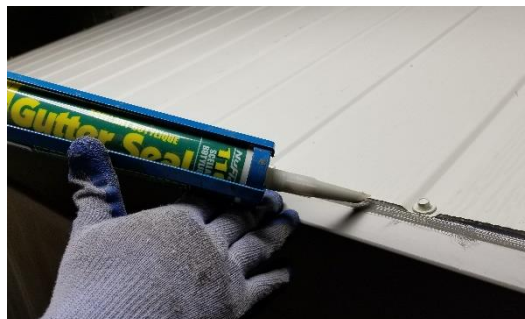
Figure 59: Sealing the roof eave kerf
