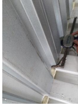
Figure 27: Panel Clamping
