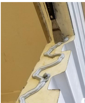
Figure 73: Serpentine bead of liquid flashing
