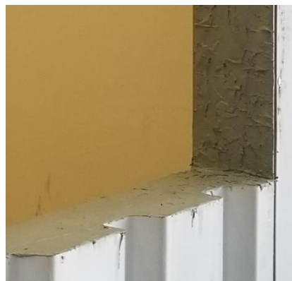
Figure 74: Properly spread liquid flashing
