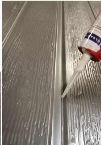
Figure 62: Applying silicone to the joint
