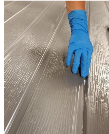
Figure 63: Working the silicone into the joint
