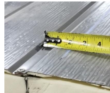
Figure 64: Snap a chalk line 2" from the seam.
