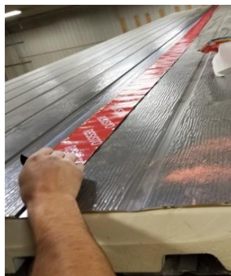
Figure 66: Aligning the barrier with the chalk line
