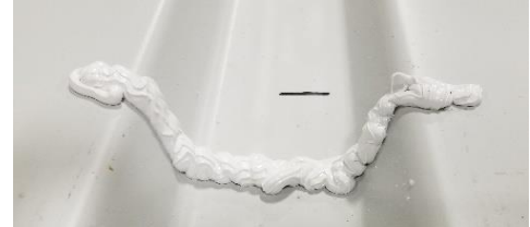
Figure 43: Foam Closures 1/2" sealant bead
