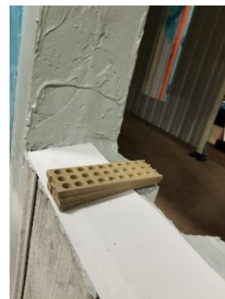
Figure 75: Shim support flashing and shims
