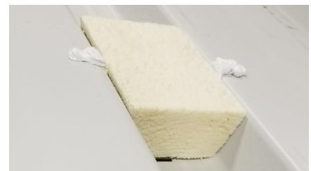
Figure 44: Installed Foam Closures
