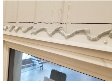
Figure 80: Serpentine bead of liquid flashing applied to drip cap
