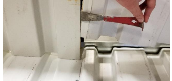
Figure 14: Trim Pry Bar used to help start inserting the tenon side into the channel side of the previous panel
