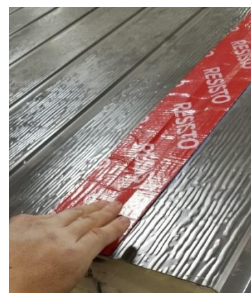
Figure 67: Applying the barrier
