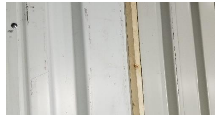
Figure 32: Shim for cut panel
