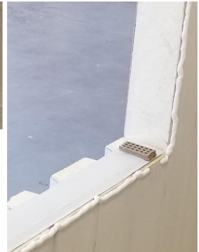
Figure 77: Sealant bead with drain gap
