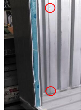
Figure 28: Screw Placement
