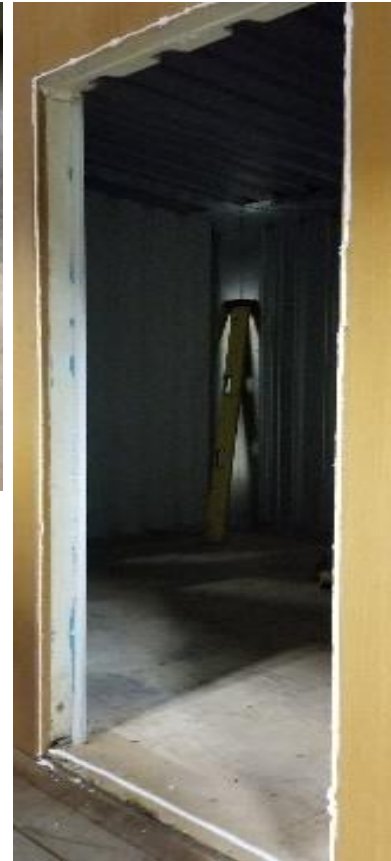
Figure 85: sealant bead around door opening
