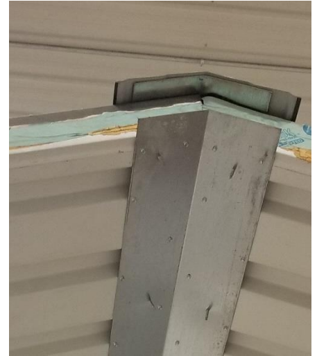
Figure 56: Ridge cap, top and bottom ridge support angles with roof panels sandwiched between
