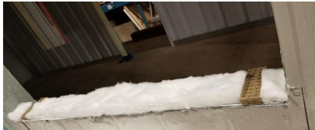
Figure 76: Fibreglass batt insulation on the sill cut to fit around the shims
