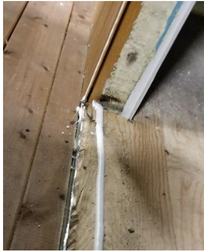
Figure 83: 1/2" bead of sealant for sealing the threshold to the floor
